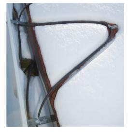
**LEFT:** Heating cables can be permently installed in walkways, but portable units can also be used to keep a high-traffic area clear at key times, such as during a move or renovations.
